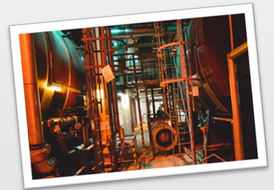
Estates refurbishment and maintenance (£8.3m)
